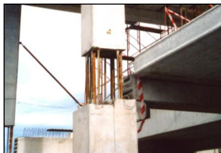
Figure 1. Steel reinforcement bars are left exposed during casting work at the factory to allow for site casting. (Courtesy of Elliott, K. S. University of Nottingham, UK.)
