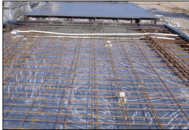
Figure 5. Electrical ducting, if required is to be installed in the precast building component prior to the casting of concrete.
