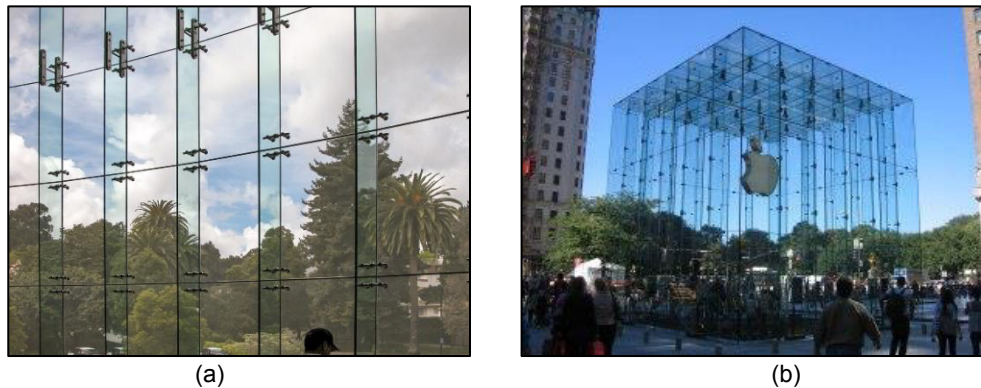
Figure 1: (a) Glass fin systems (Enclos n.d.), (b) Glass fin and mullion of the Apple Store, New York (Apple store in New York n.d.)
