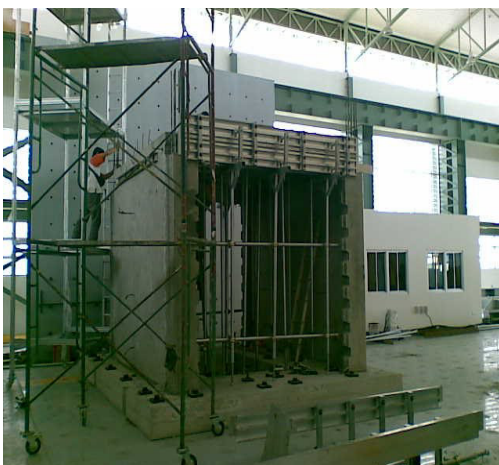
Figure 4. Cast-in-situ beam and slab are used to joint two wall panels.
