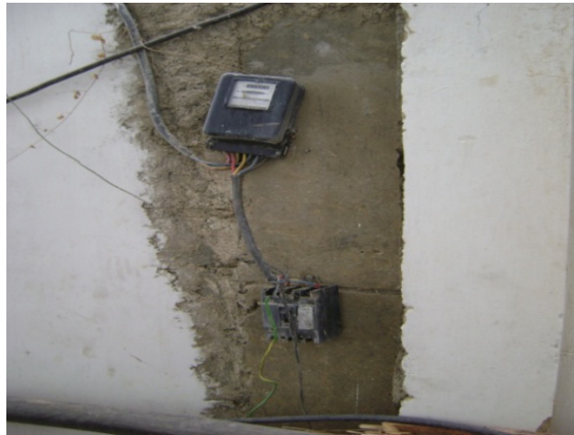
Figure 7. Unsafe electrical connections in power generation room.
