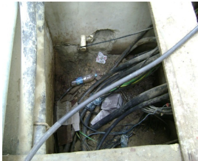
Figure 8. Electric cables trench was found uncovered. Irregular cables in trench.
