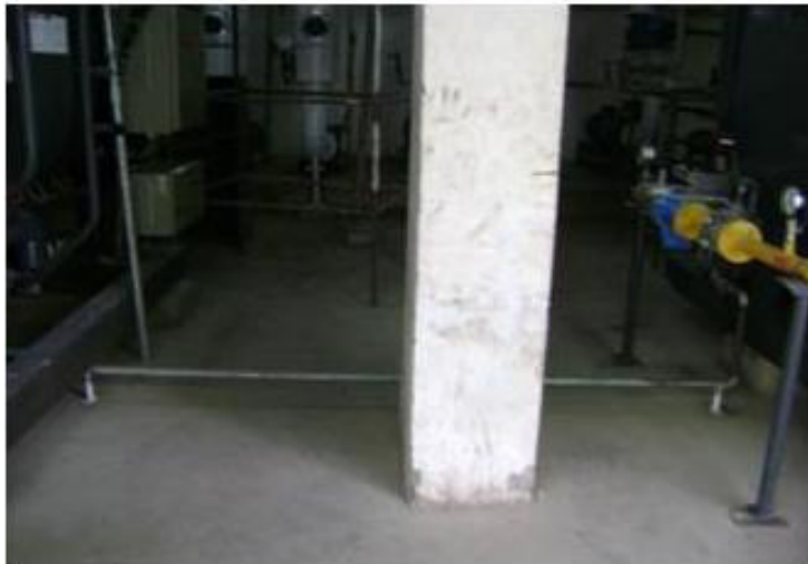
Figure 4. Diesel dosing pipe. Cause of trip hazard. Permanent design fault and cause of repeatedly occurrences of trip cases.
