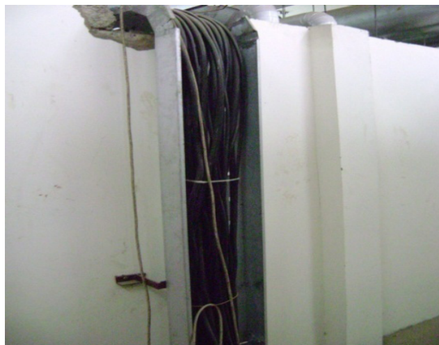
Figure 9. Uncovered electrical cable trench in power generation room.
