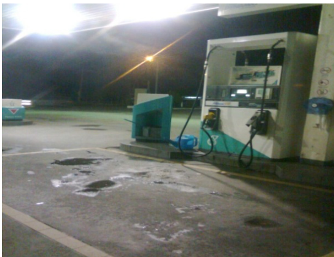
Figure 10. Spillage of petrol closer to dispenser unit at PFS.
