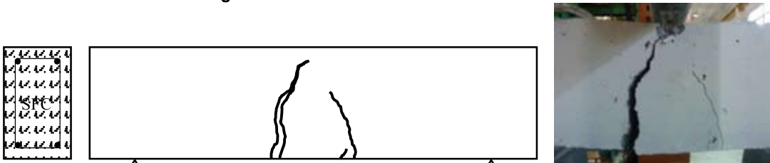
Figure 3.14. Cracks Pattern on SFRC Beam 3
