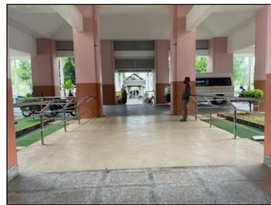
Figure 8. Ramp at Hospital B
