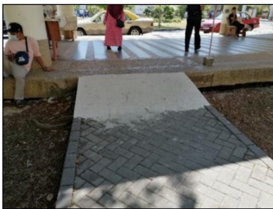
Figure 7. Ramp at Hospital A
