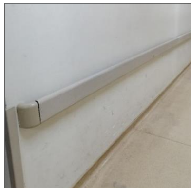
Figure 10. Handrail at The Entrance of Hospital B
