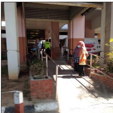
Figure 9. Handrail at Hospital A
